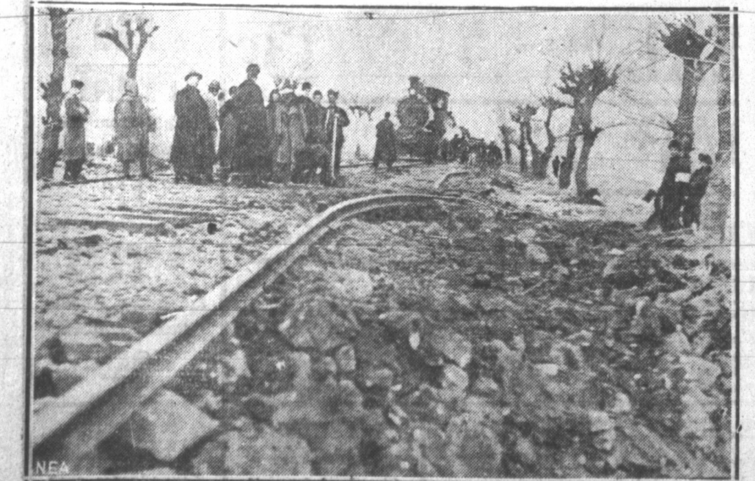
Japanese shells and aerial bombs found their mark. This picture, taken on a main line railroad near Kiangping, Manchuria, shows how the tracks were ripped up by the heavy bombardment which preceded the fall of the city. Chinese workers are shown vainly trying to repair the damage before the advance of the Japanese forces while a train waits for clear passage.
