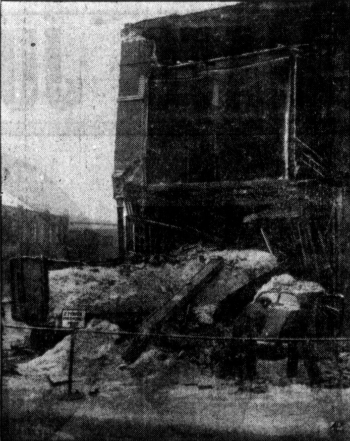
HERE'S A HOUSING PROBLEM which was quickly solved in Memphis, Tenn. A 20-foot brick wall on this vacant building at Beale and Front streets collapsed like a house of cards when rammed by a 10-ton truck and car which had collided. Two occupants suffered minor cuts and bruises.
