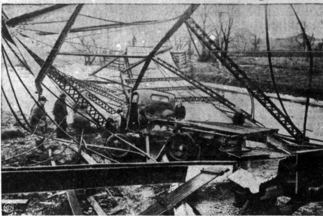
Frankfort's bridge—not London's—has fallen down and the light one and a half-ton truck, shown in the foreground of the above picture, caused it all. When the truck, driven by Landis Thompson, Sedalia, Ind., hit an end support, the entire bridge collapsed leftward. The roadway, center, shows the original line of the bridge, while the girders which formed the right side of the structure now lie across the floor and the superstructure is a mass of twisted wreckage, half submerged in the stream. The truck was damaged slightly, the driver bruised, and it will cost Indiana $20,000 to replace the bridge.
