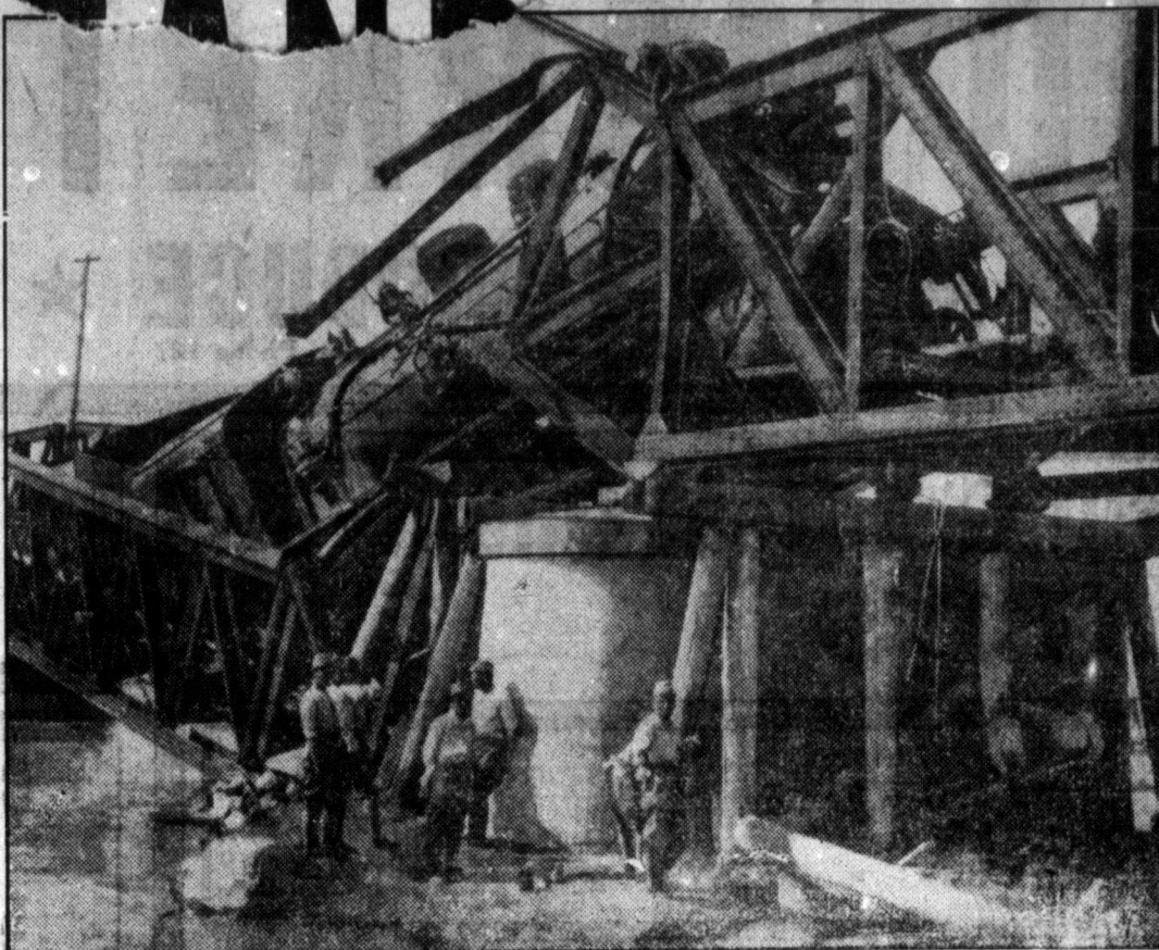
FOR PASSENGERS HERE, IT'S NO FARE because this train on the Peiping-Hankow line in China won't reach its destination. A Japanese bomb weakened this bridge and the heavy locomotive caused the structure to crumple as it rolled on. Both sides have resorted to destruction of bridges in current Sino-Japanese conflict.
