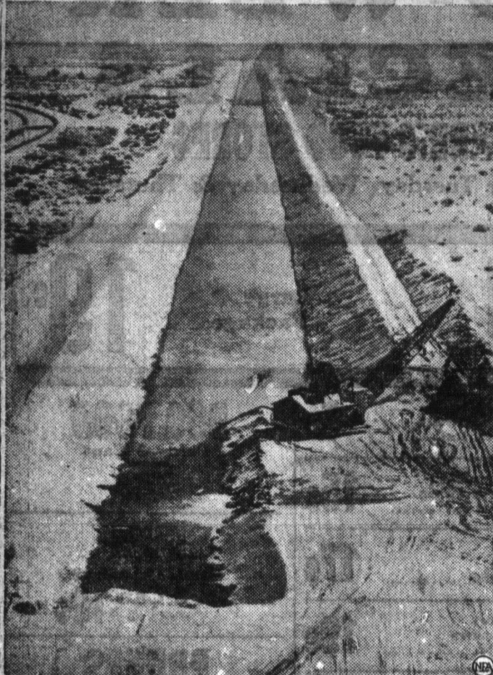
Truly a "river of life" for residents of 500,000 acres of western waste land is the now-completed All-American irrigation canal pictured above. The $3,000,000 government-financed irrigation project, largest in the world, will be operated in conjunction with Boulder Dam to control Colorado river floods and use the water to irrigate the arid Imperial Valley of California and Arizona.
