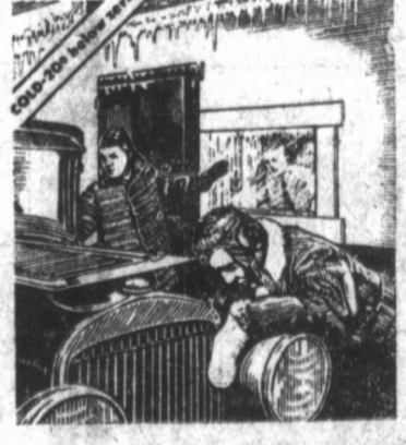
COLD-ROOM TESTS (Above right)—Here engineers reproduce driving temperatures as low as 20 degrees below zero. This verifies scientifically the "cold weather" preadjustment for Climatic Control.
