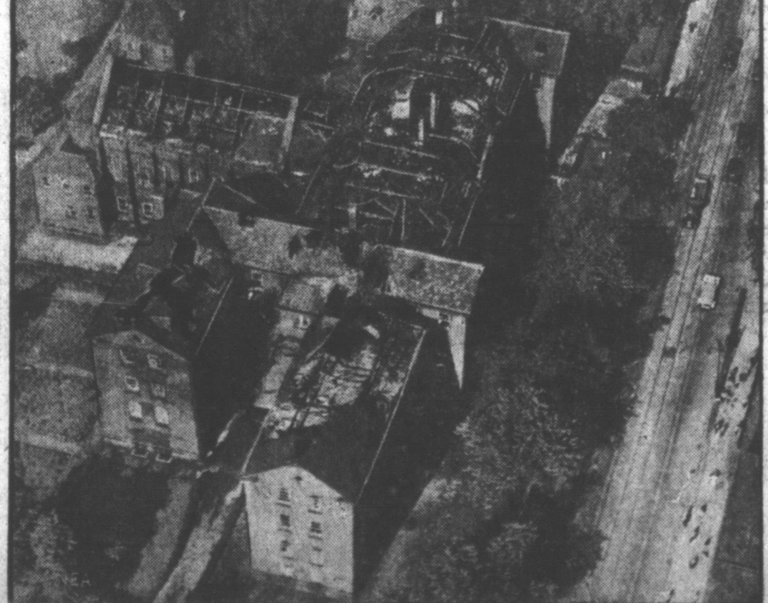
The fire-blackened ruins of the Home of the Aged of the Little Sisters of the Poor at Pittsburgh, Pa., where 26 inmates lost their lives and approximately 260 were injured when trapped in a raging fire that swept through the 55-year-old structure, are shown in this striking aerial picture. Many of the crippled and bed-ridden victims, all past 60 years of age, were burned to death in their cots.
