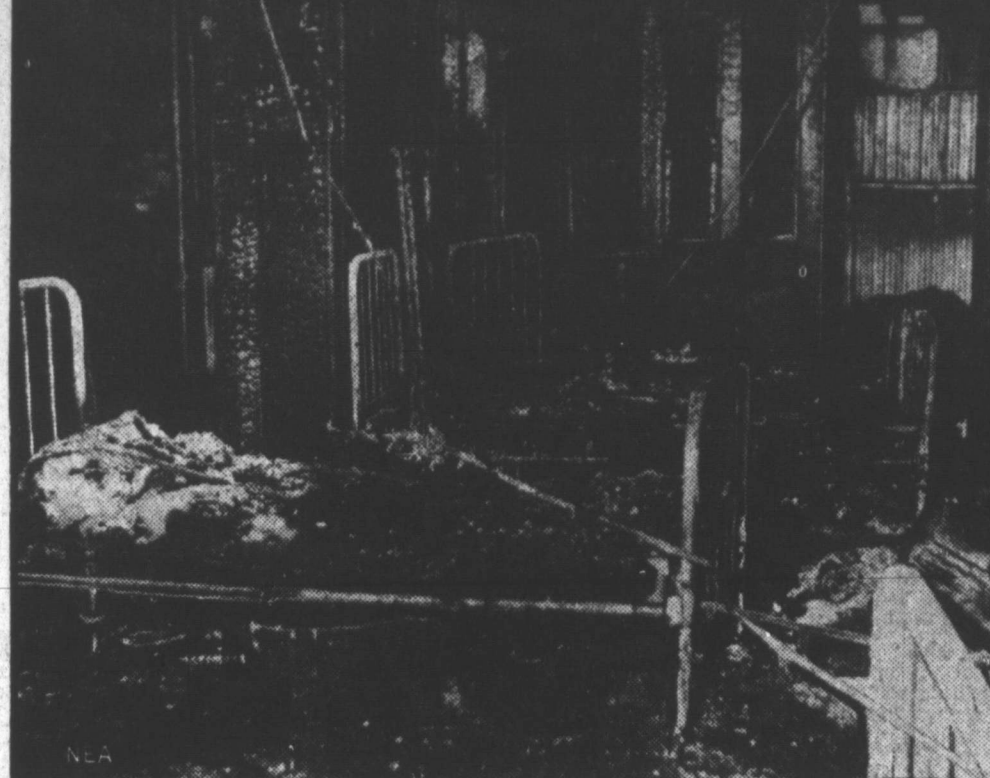
These masses of soggy blackened cloth and twisted steel are all that remained of the cots from which aged men and women tumbled, many of them to die in the disastrous fire at Pittsburgh. This picture was taken a short time after firemen quelled the blaze.
