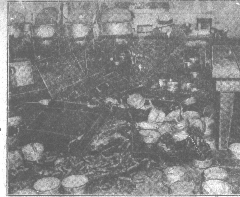
Here is how the kitchen of the antiquated state prison at Joliet, Ill., looked after rioting convicts had wrecked it during a short-lived revolt. Guards battled them for an hour, killing one and wounding three before order was restored.
