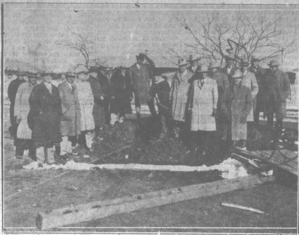
The above photograph shows the breaking of the ground for the new Gray county courthouse more than a year ago. Since the day was too cold for comfort, little more than the sod turning was done at the time.
