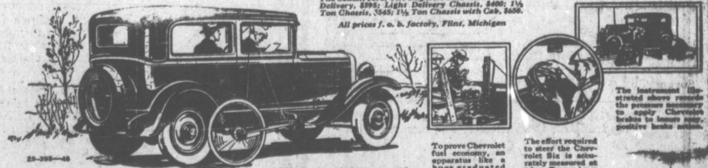
A fifth wheel speedometer accurately measures speed and mileage on all Chevrolet test runs at the Proving Ground.
