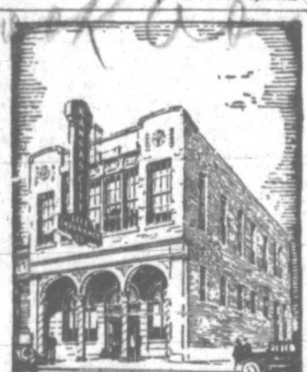
The O. Sam Cummings Agency Building, Dallas
