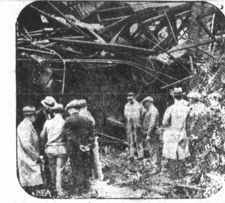
The wreckage of the plant of the Alexander Aircraft Co. in Denver, in which nine persons lost their lives in an explosion and fire, is pictured above. Four investigations are under way in an attempt to fix responsibility for the blast, which occurred in a workshop where airplane wings were being sprayed with highly inflammable lacquer.
