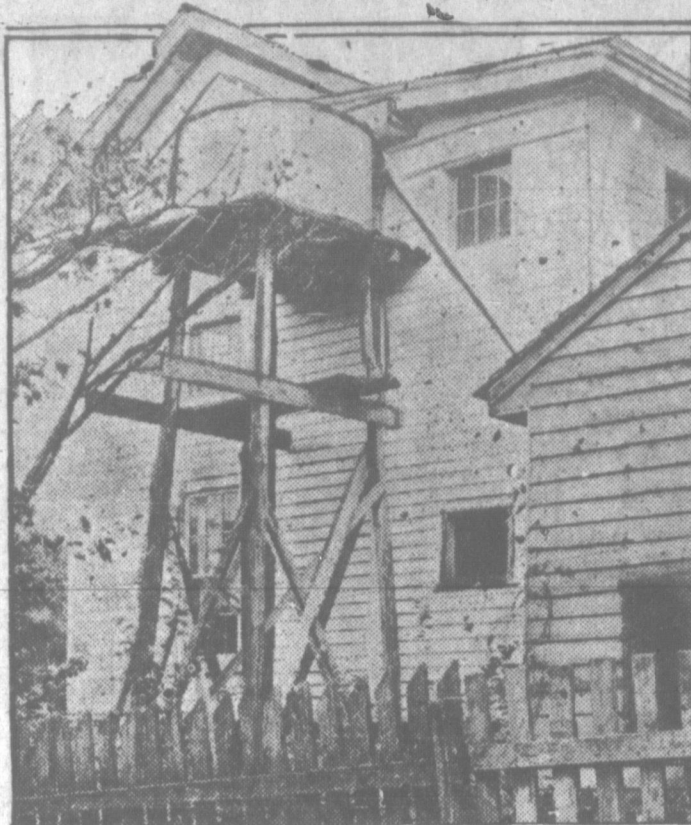
Elevated exterior tank supplies Virginia farm house with running water. U. S. V. A. Photo.
