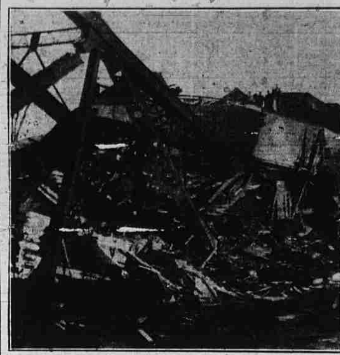
Seven cars piled up on the embankment of the Nemaha river, near Auburn, Neb., when a freight train was wrecked while crossing the stream. Note the demolished bridge. (Associated Press Photo)
