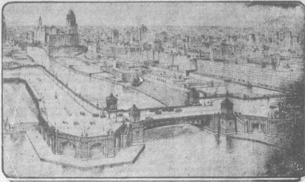
Chicago's two ribbons of lakefront highway are to be linked in the loop by a super-highway, one mile long, which will cost $10,000,000. The drawing above shows the 140 foot wide pavement, which will span the Chicago river on the loop lakefront to eliminate part of Michigan boulevard's heavy traffic burden.
