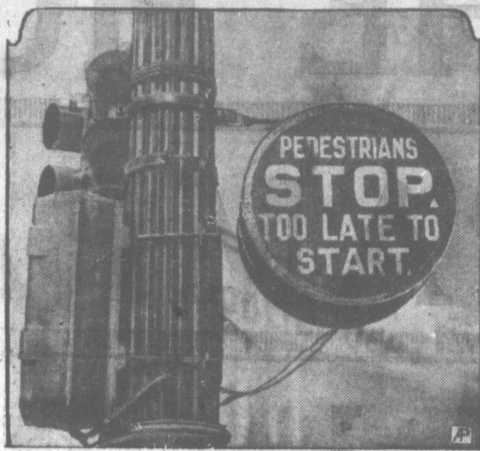
Detroit is trying out a new traffic control signal, designed to safeguard pedestrians crossing busy thoroughfares. It warns those afoot when it is too late to beat cross traffic.
