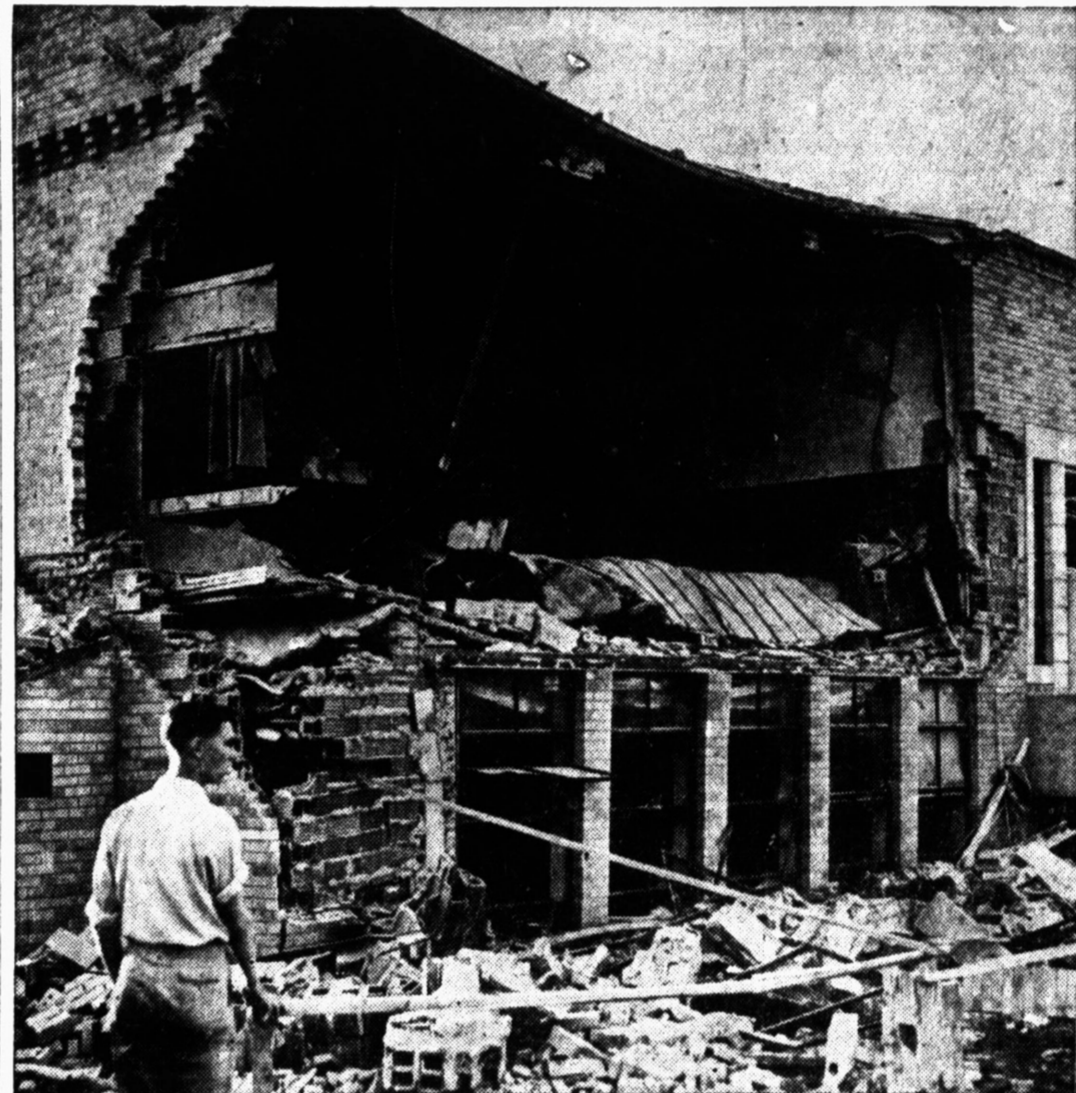
The architecture of the New London school plant and that of Pampa high school was identical, according to information received here. The explosion leveled the two wings and the front part of the building but did not completely raze the auditorium which was located similarly to Pampa's. The above picture shows a gaping hole in the portion of the structure that was not leveled. Other pictures of the explosion may be seen on page 12.
