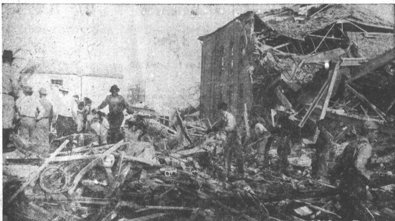
With its walls partially blasted out, one of the New London school buildings hangs precariously as
