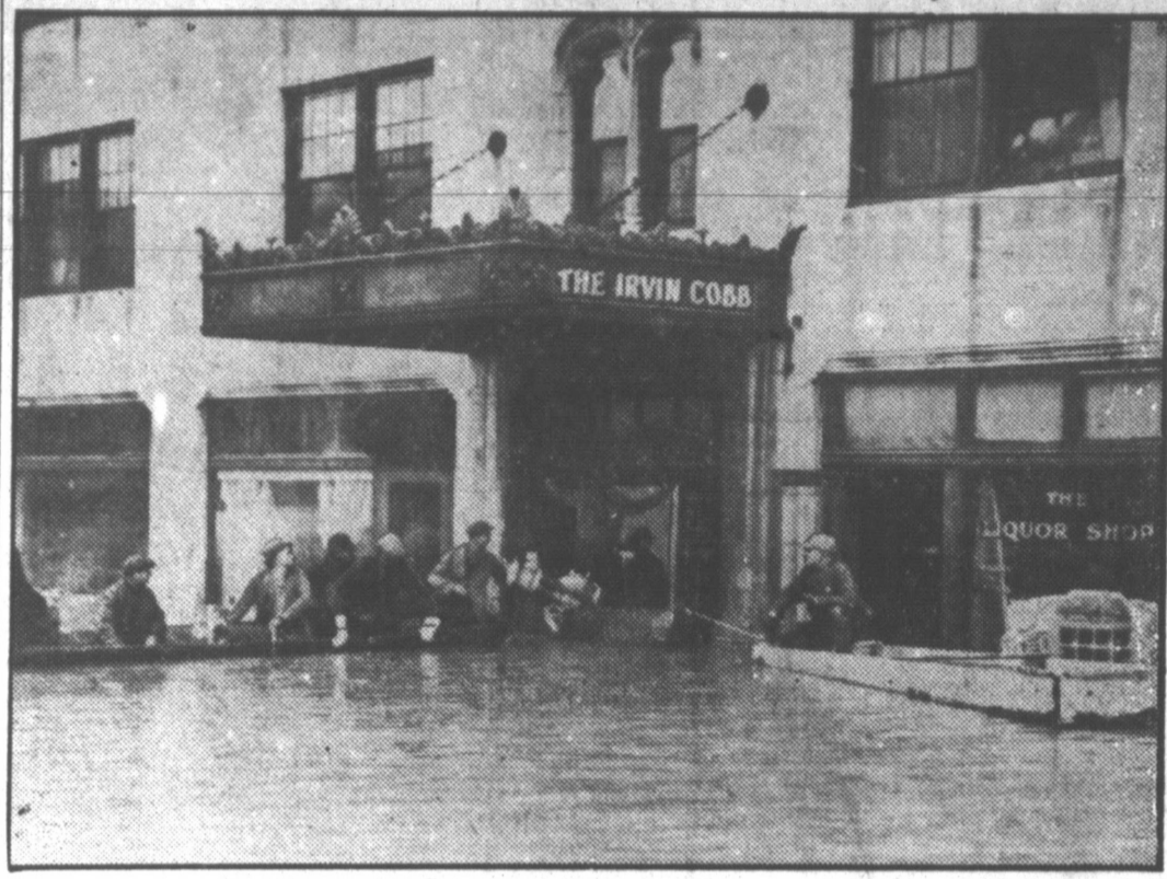
One man holds the wide front doors open and another steers the outboard motorboat right into the lobby of the Irvin Cobb Hotel at Paducah, Ky. Though the
