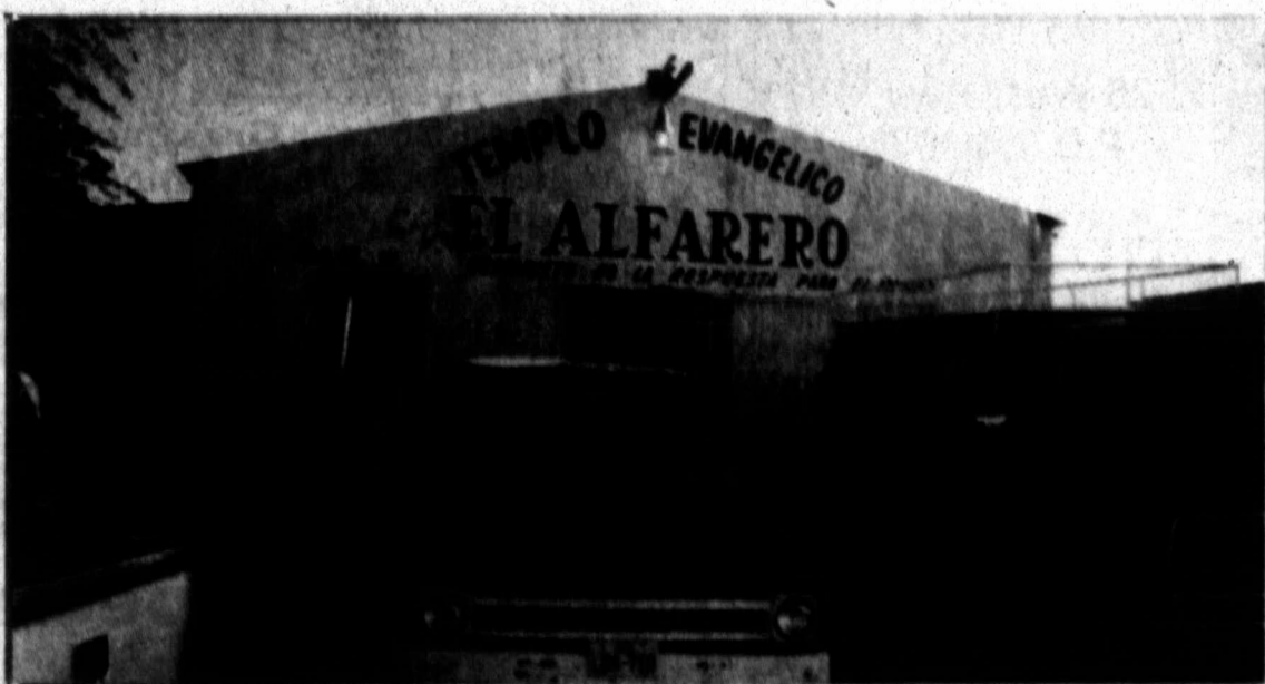
The Pampa group stayed in this church in the Mexican community while they worked to build the home for Rojelio and Gabriella. The local delegation slept in their sleeping bags as they spent their Thanksgiving holiday on the mission project.
