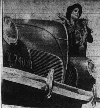
The "tear-drop" front end of the new Lincoln-Zephyr Vtype 12-cylinder cars for 1938 pictured above resembles the highly-streamlined front of a racing plane. The conventional radiator grille has been subordinated. The front is closed except for two openings near
