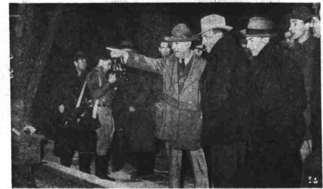
TROOPS HALT COMPLETION OF OKLAHOMA DAM—Maj. H. B. Farris of the Oklahoma National Guard points to the uncompleted gap in the Grand river dam as he discussed with I. N. Towne, construction superintendent, stoppage of work on the dam at Elmer, Okla., under martial law.
