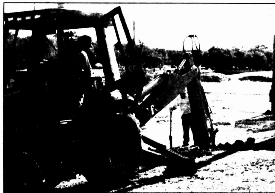
City employees Billy Jones and Peter Rodriguez dig for a water tap in preparation for Super Playground build days Oct. 21-25.
