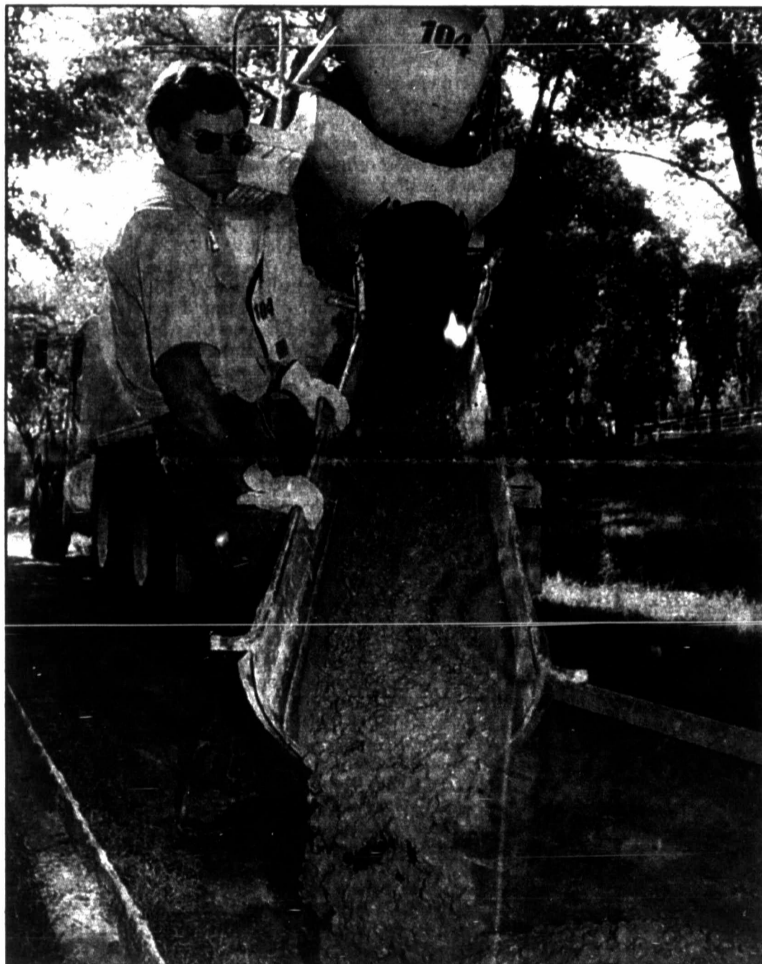
William McCarley of the Pampa Parks Department pours fresh concrete into forms along Red Deer Creek in Central Park. The concrete walkway the parks department is pouring is part of the city's hiking and biking trail system.
