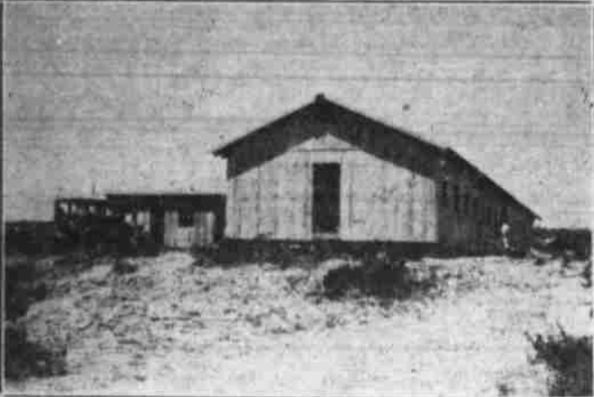
First of the buildings to go up on the permanent C.C.C. camp site here is the mess hall, pictured above. Tuesday it was all but completed and kitchen equipment was being moved in. It is here that the 234 men stationed at the camp will gather at meal time.
