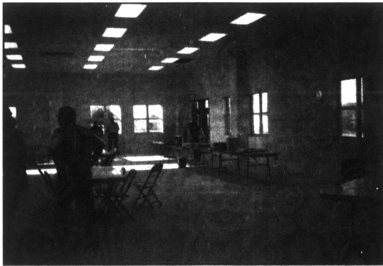
(Pampa News photo by Miranda Bailey) School board members received a tour of Lamar Elementary's new cafeteria Thursday night. Construction workers and architects showed off the remodeling being done at the school and promised school officials that construction would be finished and classrooms ready for the first day of school in September.
