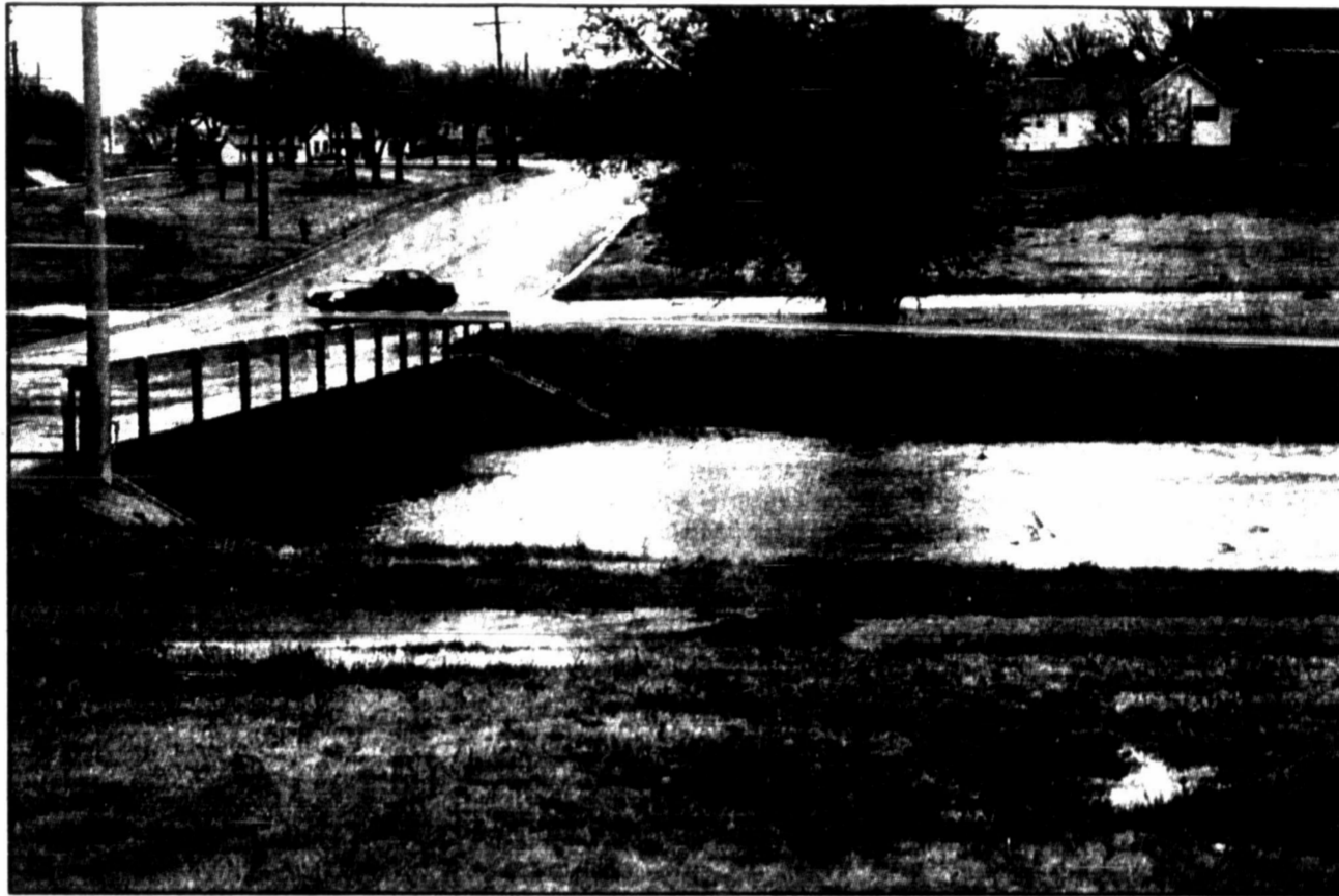
Two days ago children were walking across this nearly dry creek at M.K. Brown Park behind the municipal swimming pool. Today, after more than 2 inches of rain overnight, the creek is overflowing and the fast-moving water is near the top of the bridge. More rain is expected today and tomorrow.
