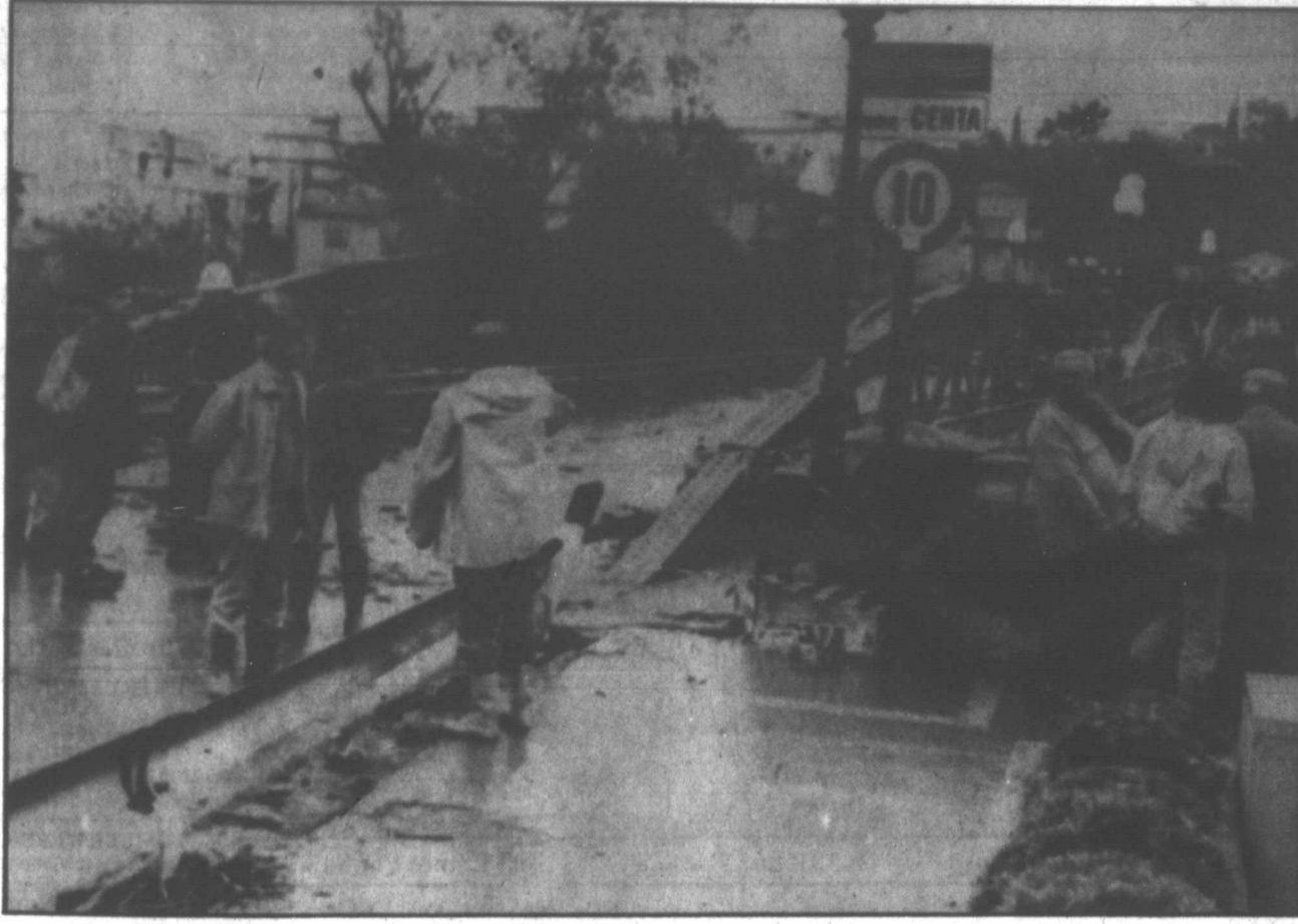
Firemen block the entrance of a bridge over the river Centa at Albenga, Italy, for fear of collapse Sunday as torrential rains swept southern Europe. (AP photo)
