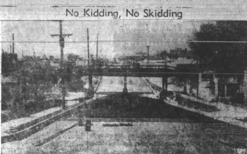
Motorists in Klamath Falls, Ore. are getting a break this winter. A snow-melting highway is being built on a steep stretch of road. Iron pipe coils, which will be heated by natural warm springs during the snow and ice season, are being installed along the highway.
