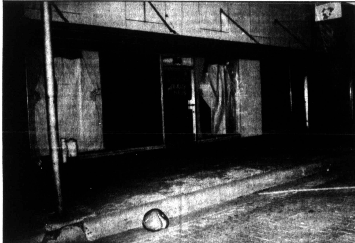
This newly installed 4 foot-by-8 foot plate glass window at 310 S. Cuyler replaces the one smashed by a pumpkin sometime Saturday night or Sunday morning. An estimated $300 damage was caused. No injuries were reported. (Pampa News photo by Cheryl Berzanskis)
