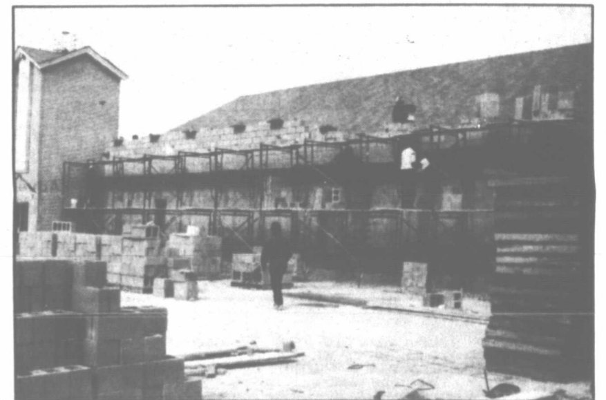
Construction progresses on Central Baptist's educational building. (Special photo)
