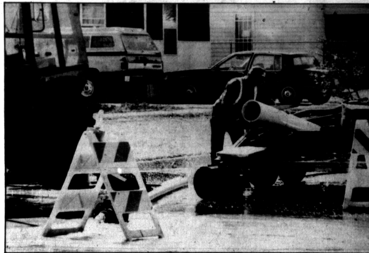
City crews work this morning on a water line leak at Gillespie and Foster. During the repair work, water from the line flooded down the street while the crews blocked off the area to complete their repairs. (Pampa News photo by Danny Cowan)
