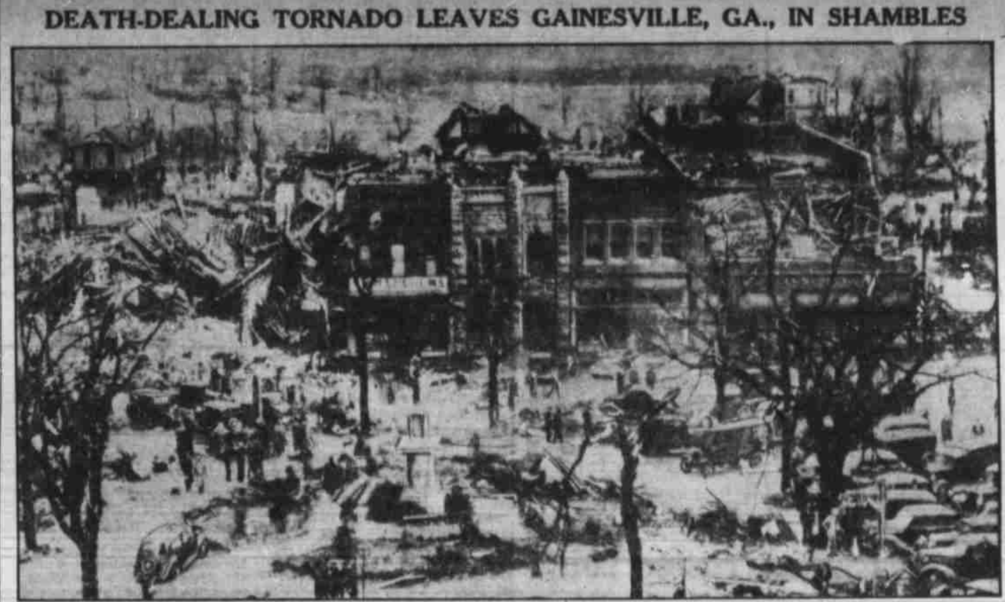
This graphic Associated Press photo tells a terrifying story of death and misery which haunted Gainesville, Ga., after a tornado reduced the town to debris. The picture shows a general view of the area in which approximately 200 persons were killed and hundreds injured.
