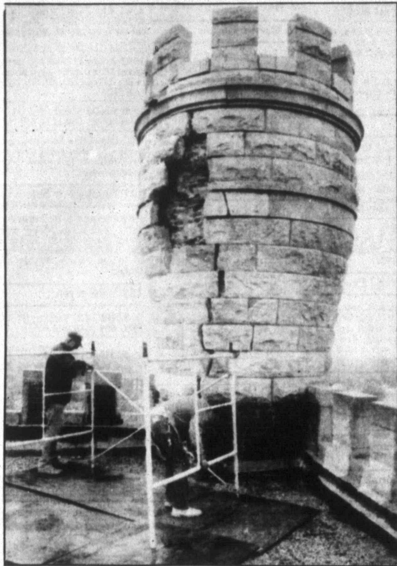
Eastern Illinois University officials assess lightning damage Wednesday to the campus Old Main building in Charleston, Ill. A turret in the center section of the building, which resembles a castle, was struck by lightning during a storm Tuesday night. The jolt blasted stone facade from the turret and widened a crack in the century-old structure. (AP photo/Charleston Times Courier)
