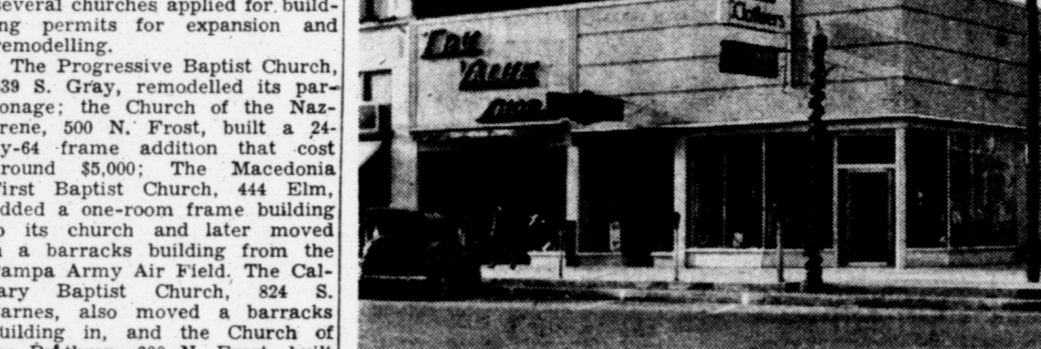
ANOTHER new building changing the face of downtown Pampa is this new building at the corner of N. Cuyler and Francis, built this summer for the Roy Van Vliet interests of San Francisco. It is now occupied by the S&Q men's clothes, Mode o' Day, Tru Value Shop, and Coston's Bakery.
