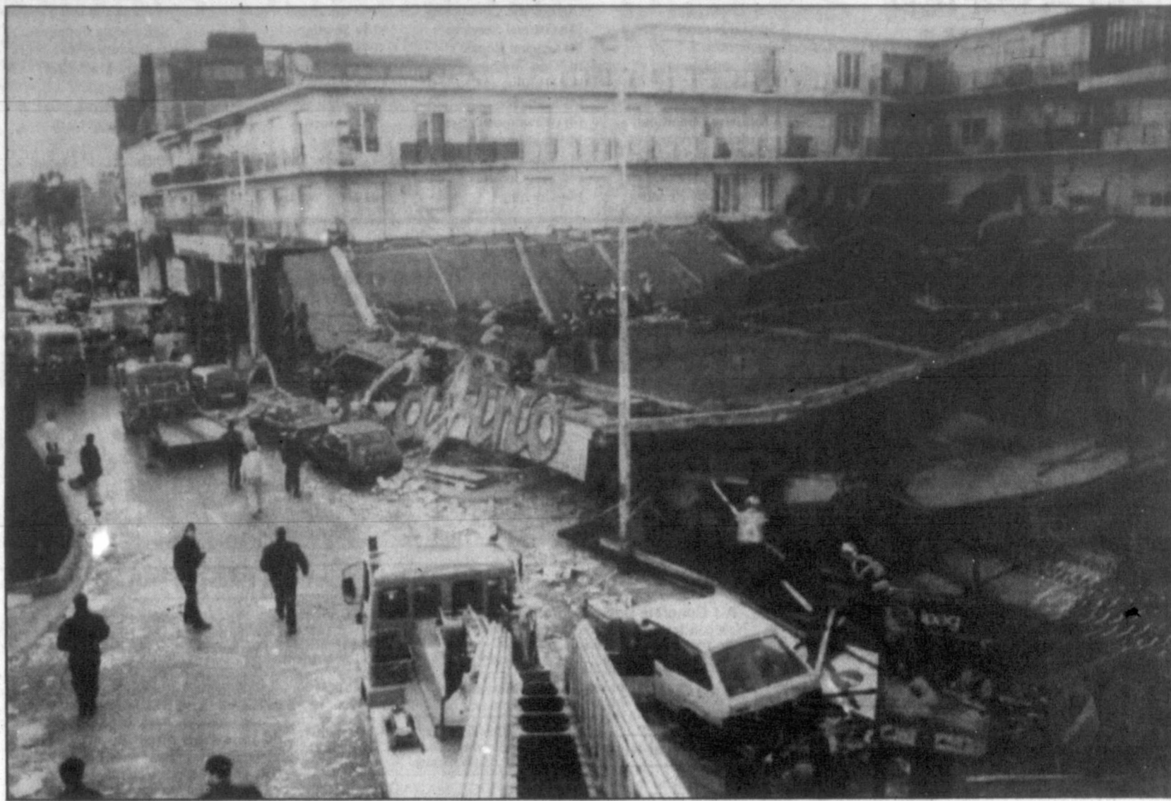
The concrete roof at a busy supermarket in Nice, France, collapsed Wednesday. Authorities said at least two people were killed, more than 90 were injured and about 15 were still trapped in the rubble. The regional civil defense headquarters had earlier reported 10 deaths, but later revised the figure. Rescue crews, assisted by dogs, searched carefully into the night, working around chunks of concrete
