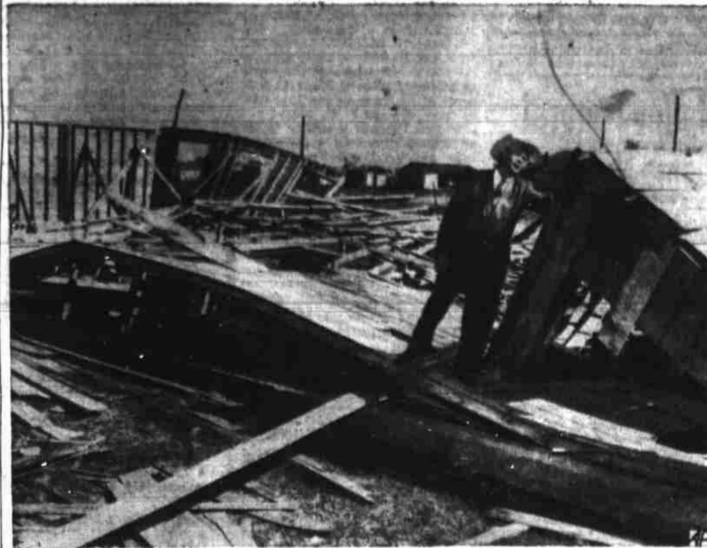
WIND BLEW DOWN CHURCH—The Rev. B. E. Smith stands amid the ruins of the First Baptist Church of Elam, a small community near Dallas, Tex. A strong gust of wind blew down two walls and the roof structure which the 150 members of the church built by working nights. They expected to occupy the church in two months. (AP Photo).
