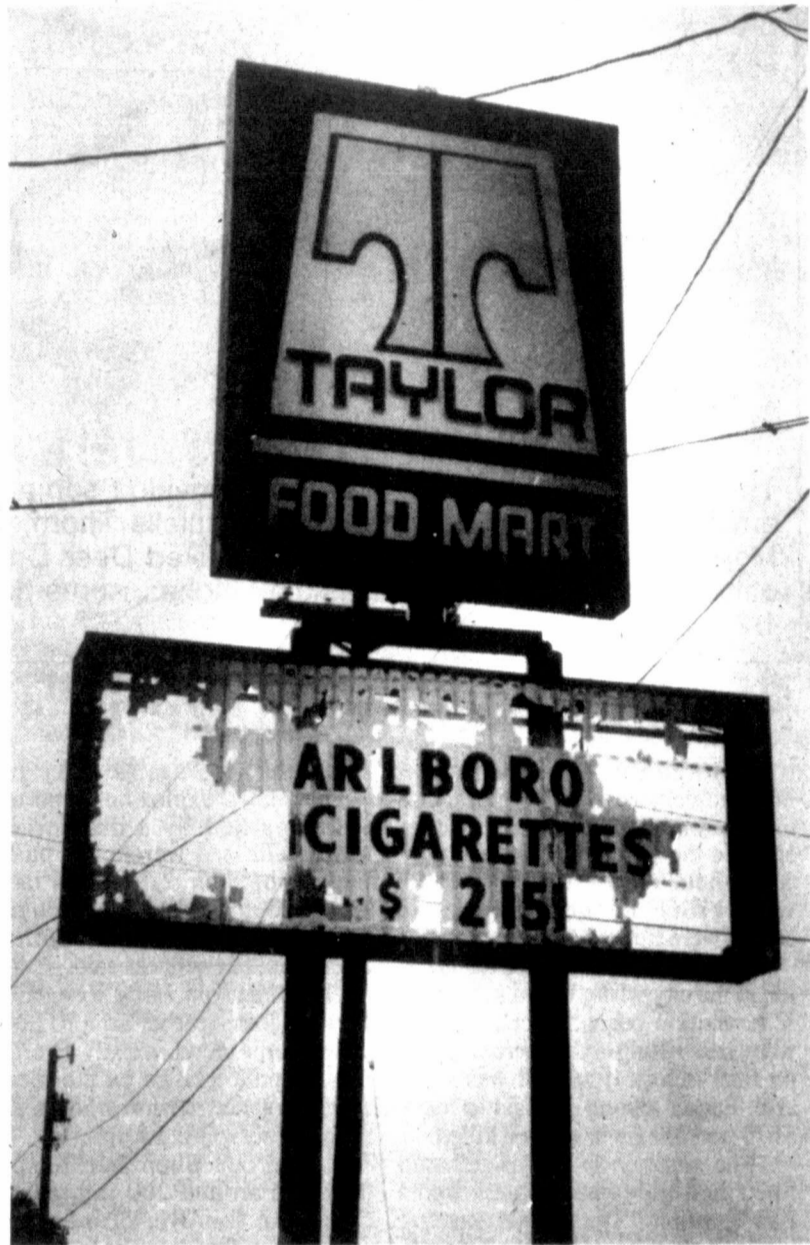
(Staff photo by Randal K. McGavock) This convenience store sign is just one of the many Skellytown structures damaged in Thursday's hail storm.
