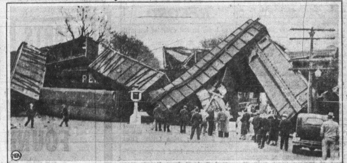
This shattered heap of boxcars provided a new and astonishing peril for motorists when a New York-Chicago freight train of 24 cars was derailed on a Plymouth, Ind., viaduct. One boxcar landed exactly on the spot from which a motorist frantically backed away as he saw the train leave the rails. Four more cars crashed down on the opposite side of the trestle within six feet of other autos halted by a traffic light at the viaduct. No trainmen were injured, though 1000 feet of track was torn up in the derailment.
