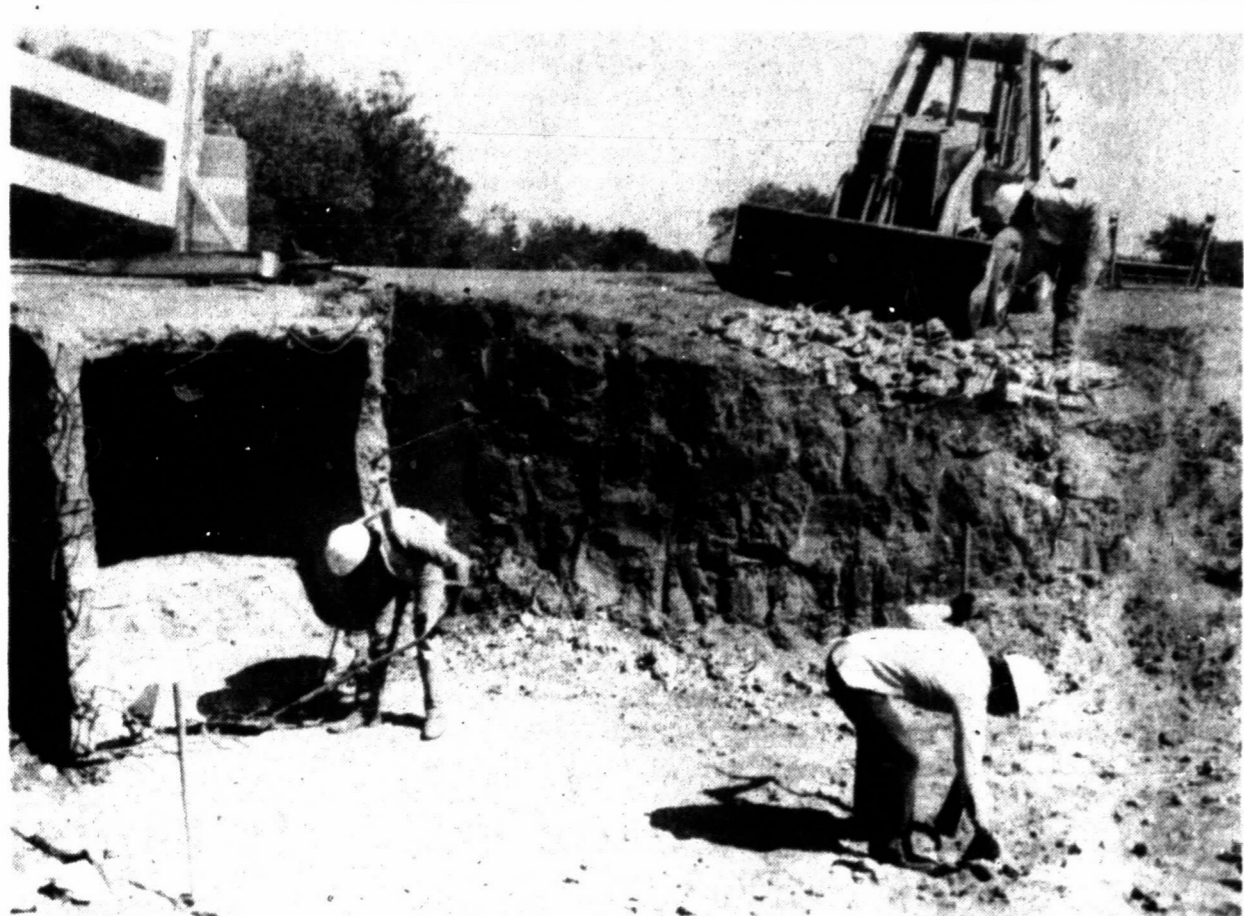
From left, Marcelin Dominguez, Hector Marquez, and Ancelmo Villa with Strickland & Knight Inc. pick up pieces of concrete and prepare a culvert to be repaired on U.S. 60 in Roberts County Thursday.
