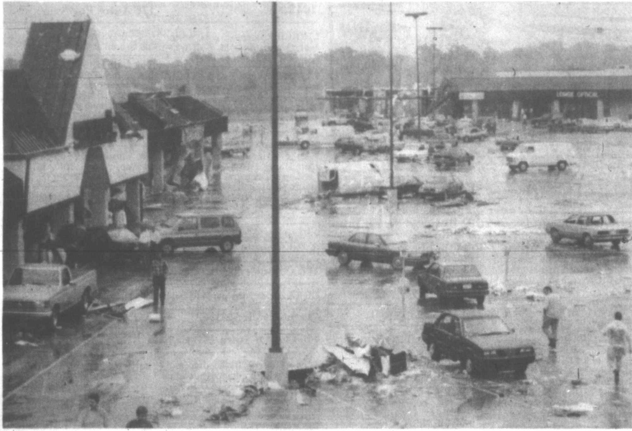
The parking lot of Fairview Shopping Center east of Kendallville, Ind., is littered with debris and overturned vehicles in the wake of a tornado that struck the town Tuesday afternoon.
