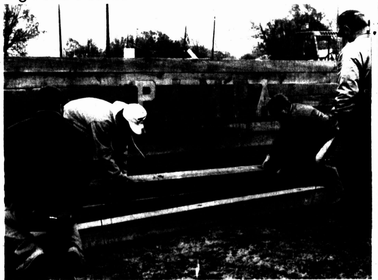
Panhandle Industrial employees, from left, Paul Searl, David Hopson, David Caldwell and Ed Taylor fix timbers at the site of the west entrance to Pampa on Saturday. The "PAMPA" sign in the back, made of aluminum, was designed and placed in the timbers by Panhandle Industrial for the Clean Pampa Inc. beautification project. Landscaping is also scheduled to be completed at the site on U.S. 60.
