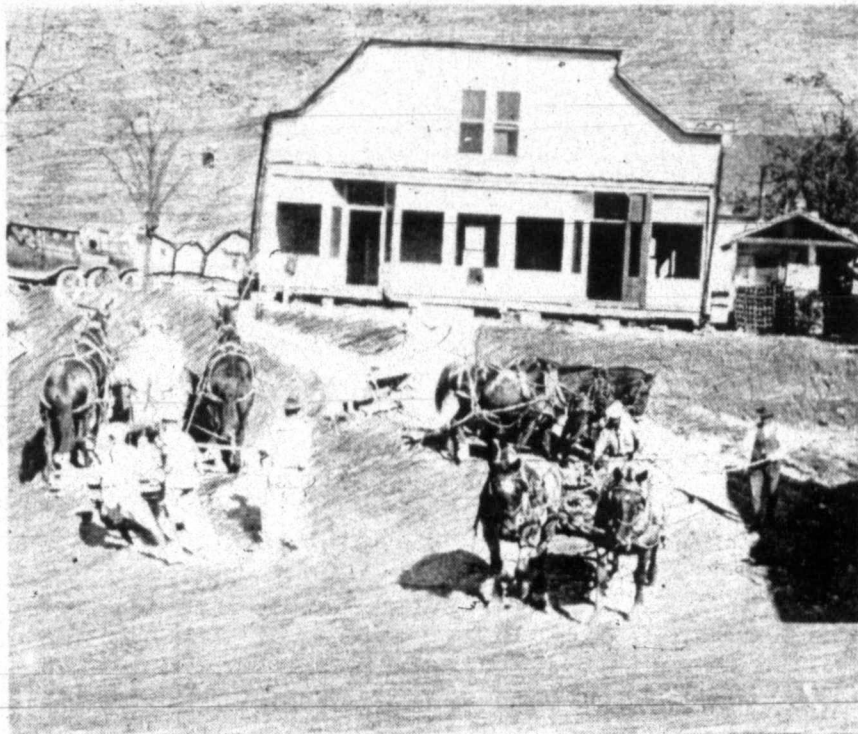
The original Brunow house at 101 S. Cuyler was moved in 1926. The false front was removed so that the house appeared smaller when it was relocated at 825 W. Kingsmill.
