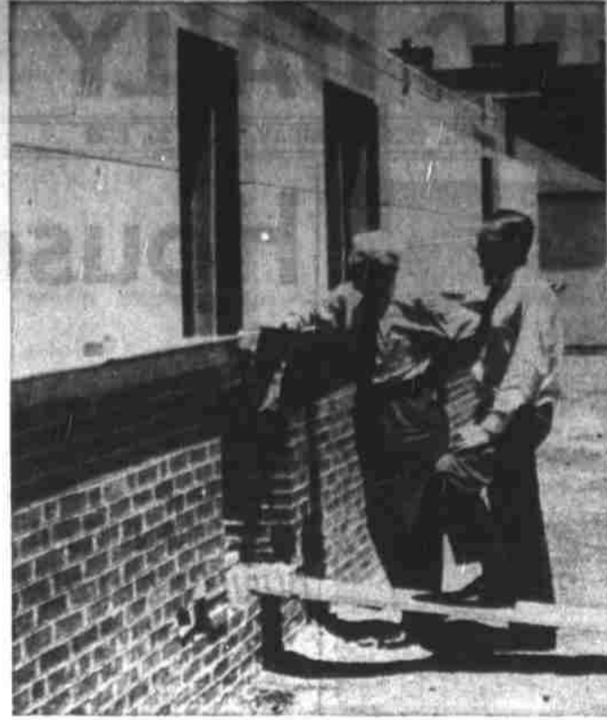
County Judge Sam Bullock left and Sheriff Dick Gregory look over the new Mitchell County jail, expected to be completed early in the fall. In the background, the old jail, built of native sandstone blocks in 1915.
