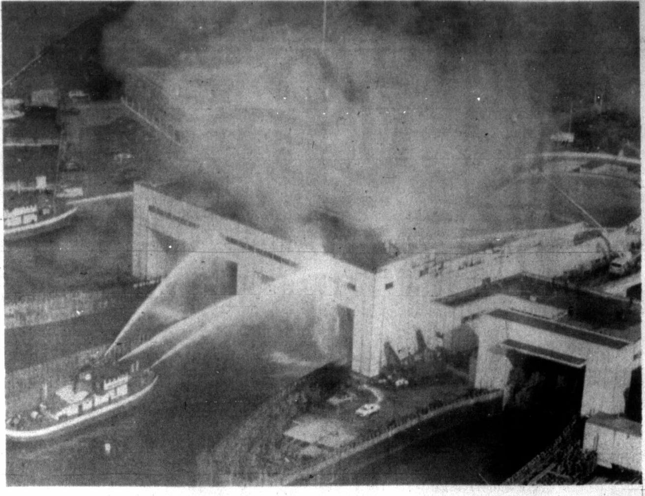
Fireboats at the Staten Island Ferry terminal in lower Manhattan douse the flames of a fire there Sunday morning. The blaze, labeled as suspicious in origin, concentrated under the terminal roof, resulting in a partial collapse and at least 13 minor injuries.
