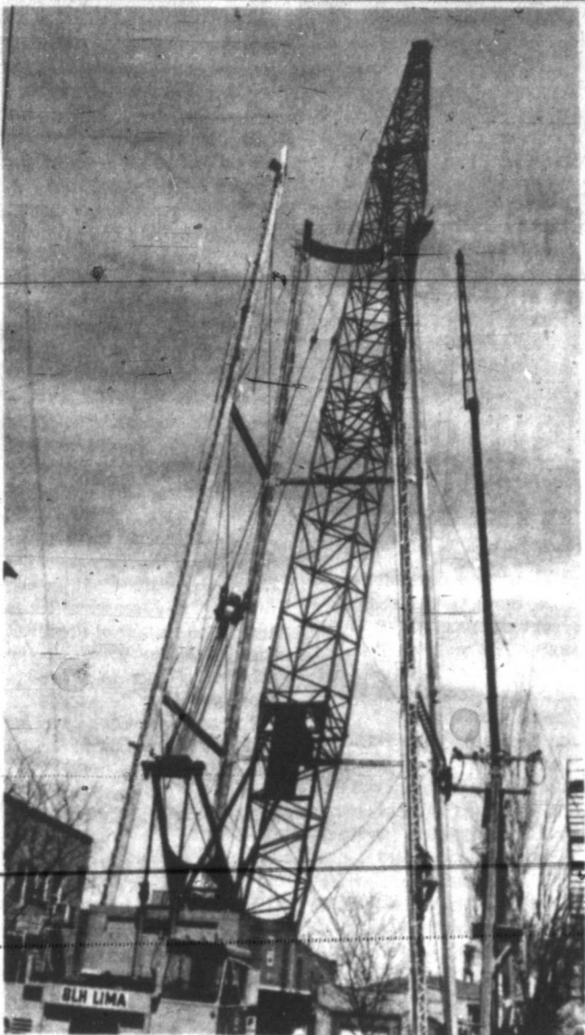
DOWN AND DOWN IT GOES—Workmen had a busy day yesterday as they removed the legs of the old water tower behind the fire department in downtown Pampa. Using giant cranes to hold the legs steady, the workers used torches to cut the legs loose before they were lowered to the ground. All that's left of the old landmark now is a few foundation moorings. (Staff Photos By John Ebling)
