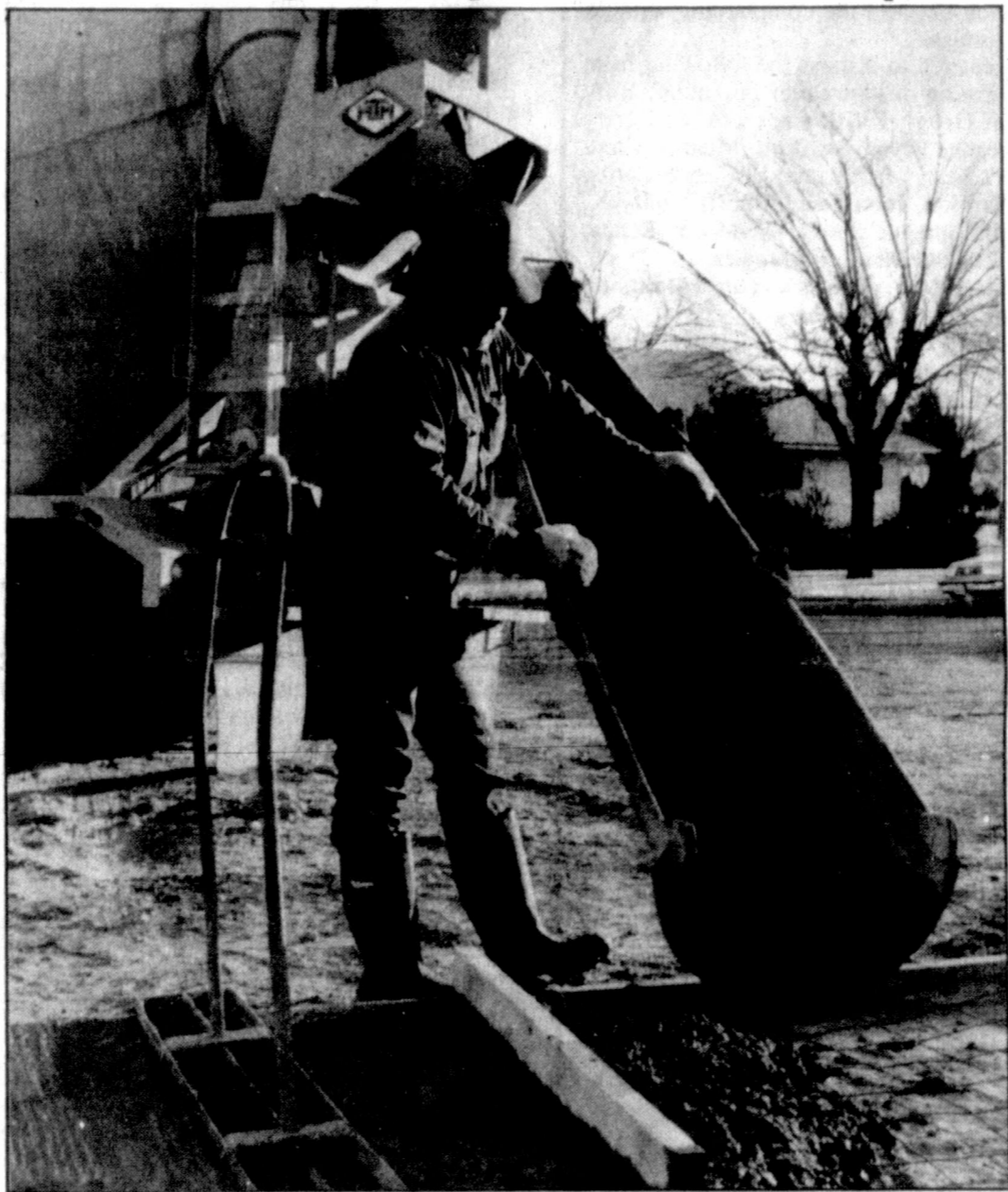
Jim Benton adds to the concrete relationship between Genesis House and the outside world today as he pours a new sidewalk to the community service agency in the 600 block of Buckler. (Pampa News photo by Darlene Holmes)
