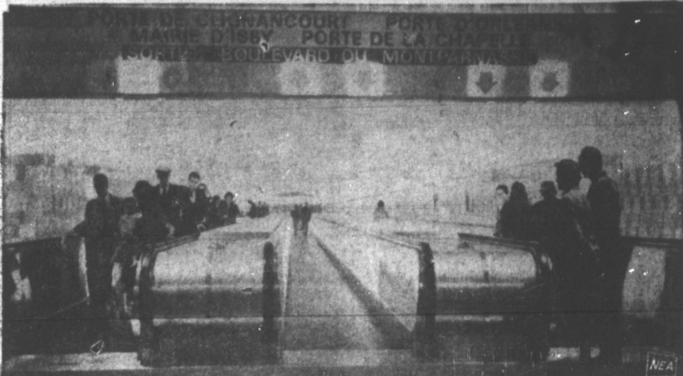
TIRED FEET get a break in Paris where Metro passengers can ride the 600-foot-long Sandvik Movator, a moving sidewalk, reportedly Europe's largest, installed at the Montparnasse-Bienvenue station.
