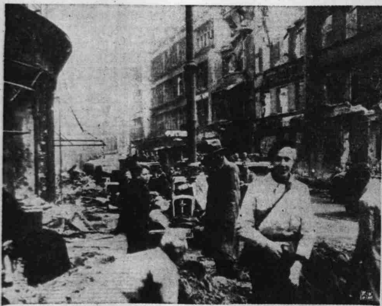
GERMANS BEGIN CLEANUP OF BERLIN WAR DAMAGE — German civilians, including women, man shovels as work of cleaning up widespread damage to the city of Berlin gets under way. Bomb-damaged vehicles still line the streets. This is Unter Der Linden in the heart of the capital. (AP Wirephoto from Signal Corps).
