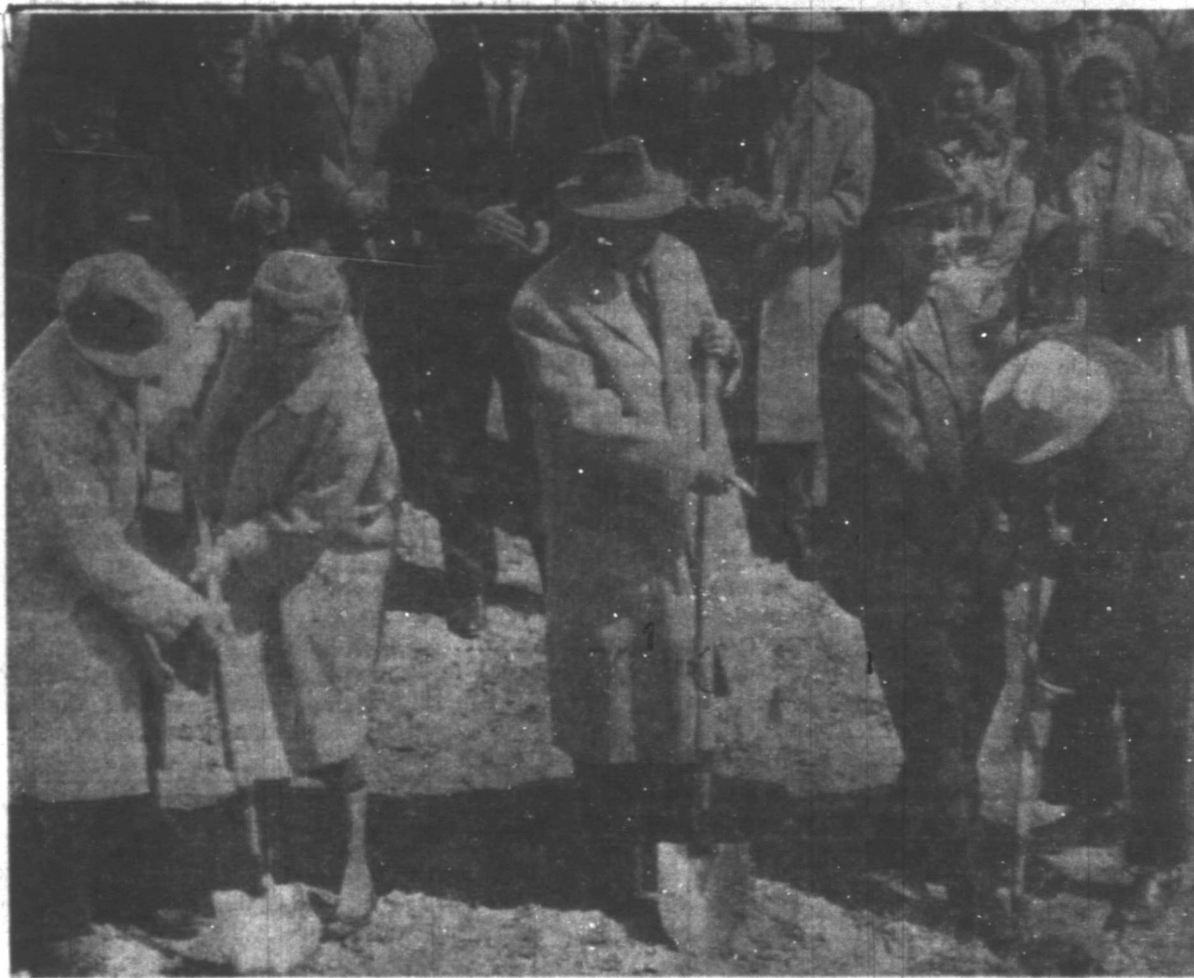
THEY 'DIG' CORONADO — It was on a chilly day in April of 1959 when these Pampa citizens broke ground and dug first dirt on the site where the Coronado Inn, a chamber of commerce and community project, stands today. Left to right in that picture taken more than nine years ago are the late C. P. Buckler, Mrs. Inez Carter, George B. Cree Jr., president of the Hotel Corp.; Mayor Ed Myatt and Warren Hassee, chamber president.
