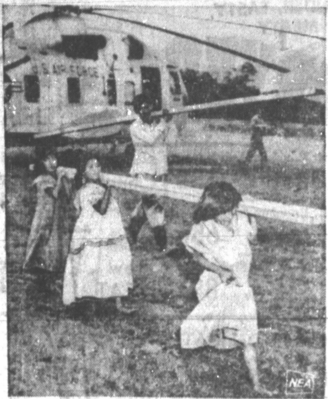
CHILDREN HELP unload lumber from a helicopter at an Indian village in Panama. In this case the building material was for construction of a medical center. It takes two days to reach the village by horseback from the nearest town, so Air Force airlifted 26 tons of CARE supplies.
