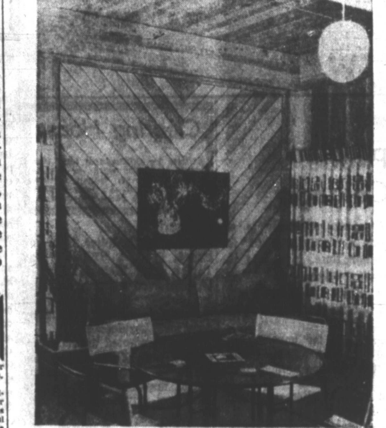
In this "rec" room, warm atmosphere and low upkeep were achieved by paneling walls in clear finished cedar. Most boards are random-length, installed vertically, but one wall is arranged in chevron pattern as accent for conversation corner and game table.
