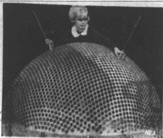
SUPERSTRAINER is really an eight-foot-diameter radar antenna. Protruding rods, like those held by Joyce Melkey, are energy feeds that will extend from each of the more than 16,000 holes in the scaled-down prototype.
